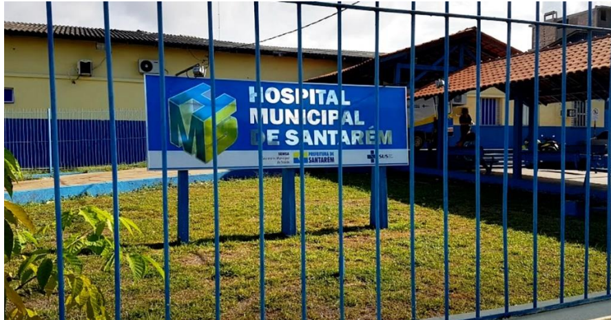
Figura 6: Hospital Municipal de Santarém
